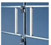
The locking wedges of the guardrails sit tightly, stiffening the rails and enhancing the feeling of security in the scaffolding.
